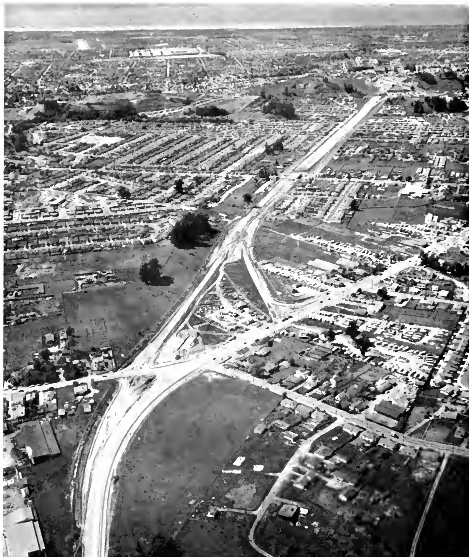
Construction on US 50 in Castro Valley; Coastro Valley Boulevard, the existing highway route, is shown to the right of the direct alignment of the freeway bypass
